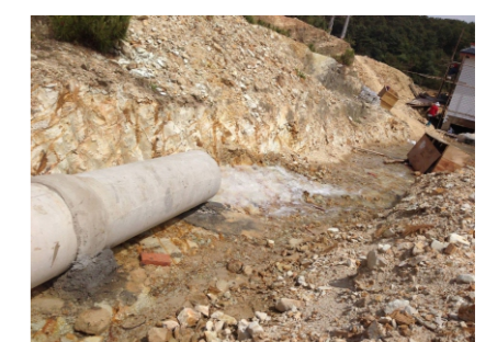
Yemen 75kw Pumping system
